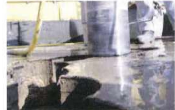
6 ..... of concrete being removed by .....
